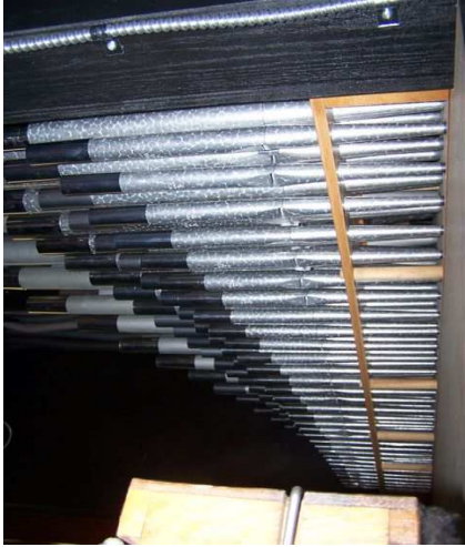
Ranks of Pipes
